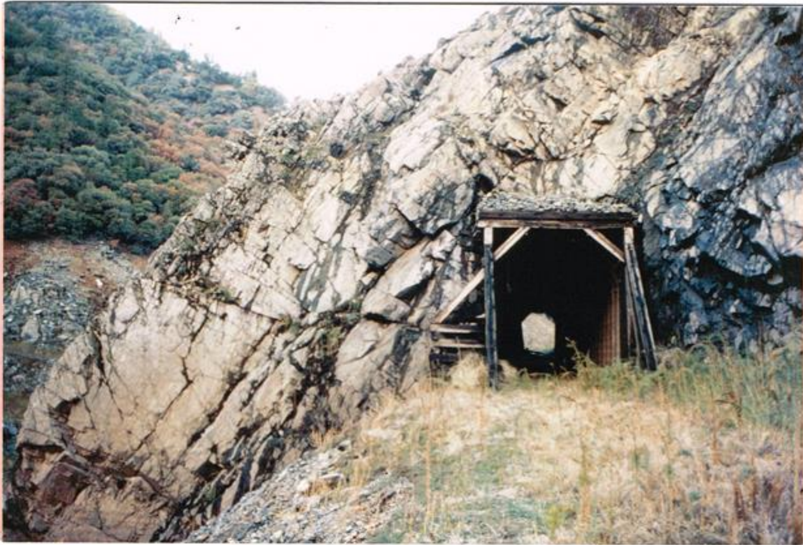
Tunnel #8 11-5-1977 Mile Post 226.9 K. Meeker
