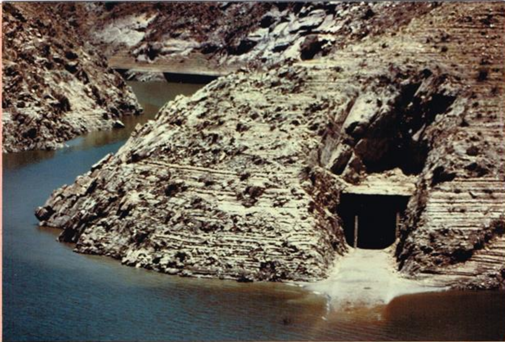
Berry Creek Tunnel #6 June 1977
