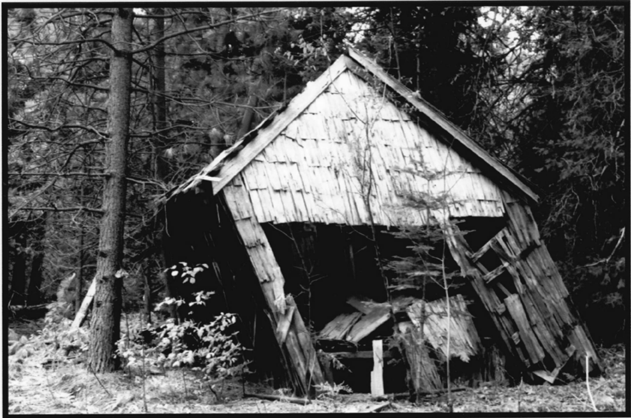
Duensing/Campbell Cabin built sometime after 1919
