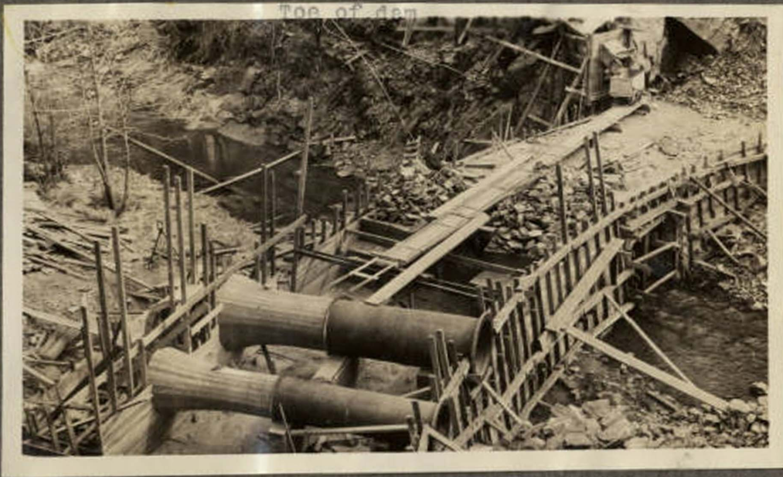
1924 Concow Dam Scrapbook Image 13b Caption: Toe of Dam
