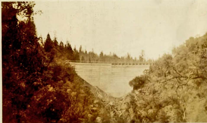
Concow Dam as seen from County Road.
