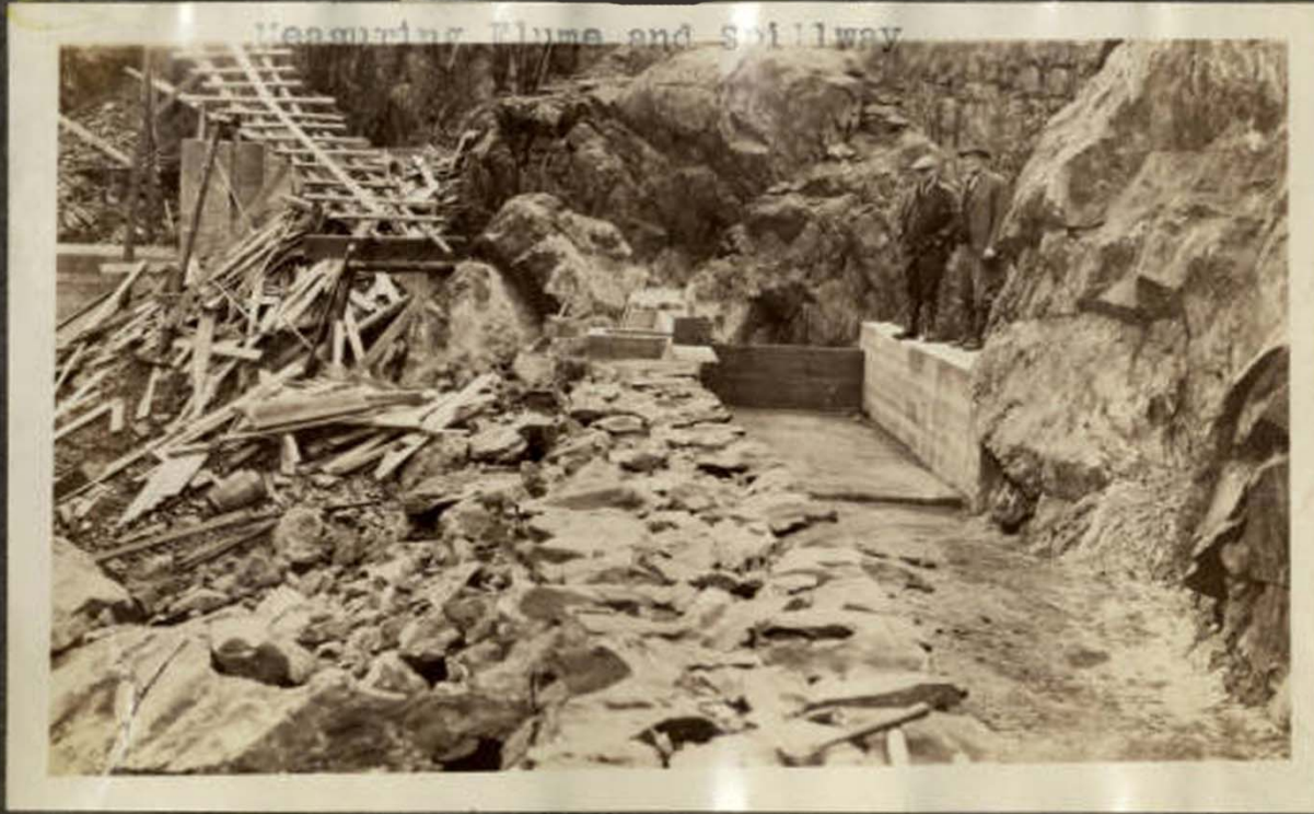
1924 Concow Dam Scrapbook Image 27c Caption: Measuring Flume and Spillway
