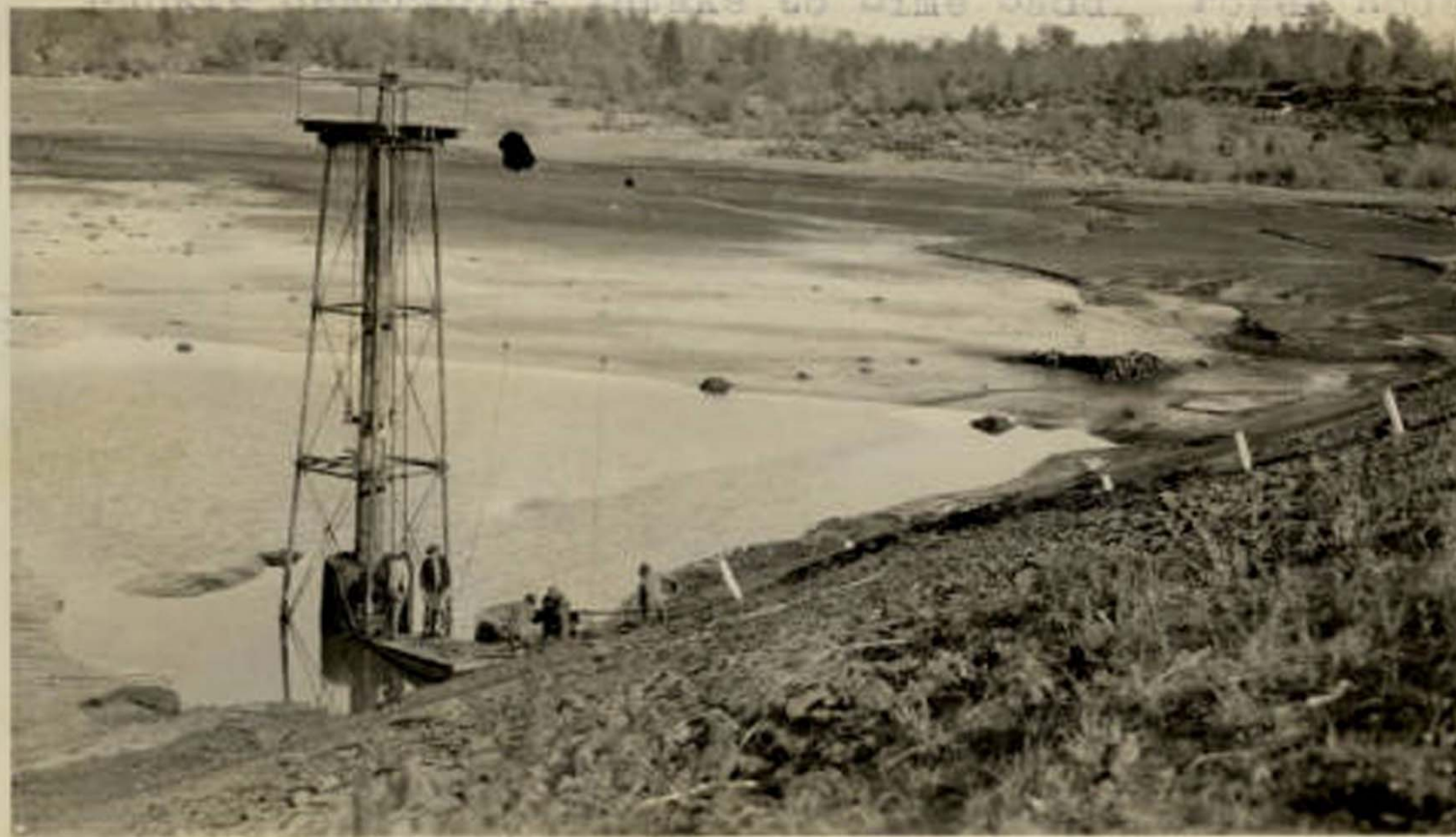
1924 Concow Dam Scrapbook Image 34b Caption: Kunkle Reservoir - Intake to Lime Saddle Power House
