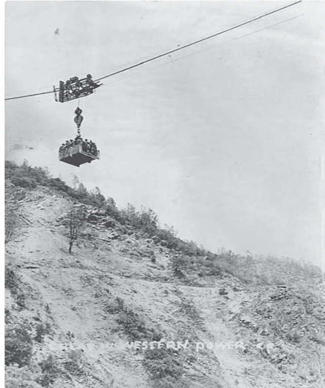
In 1908 they used an overhead tram to cross the Feather River from the town of Las Plumas to the power house on the opposite bank
