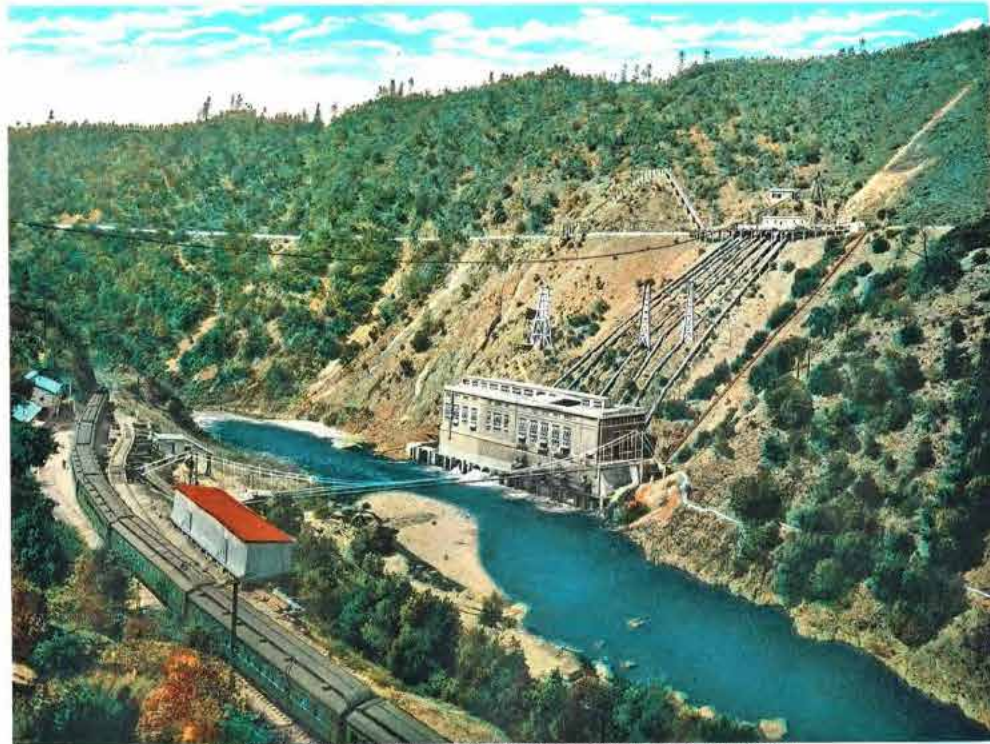
"LAS PLUMAS PLANT" GREAT WESTERN POWER COMPANY OF CALIFORNIA.
