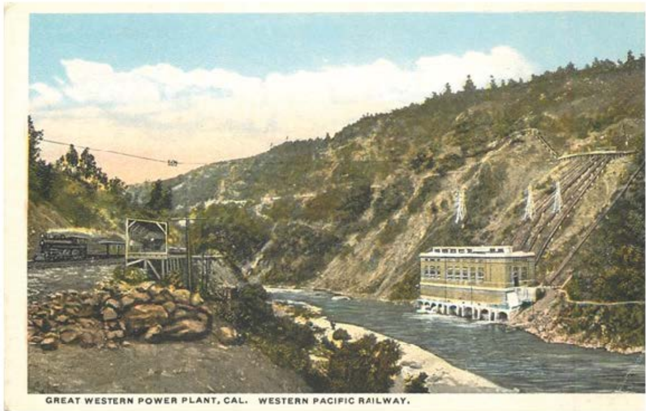
Las Plumas Power house circa 1920 after 1912 expansion on far end.
