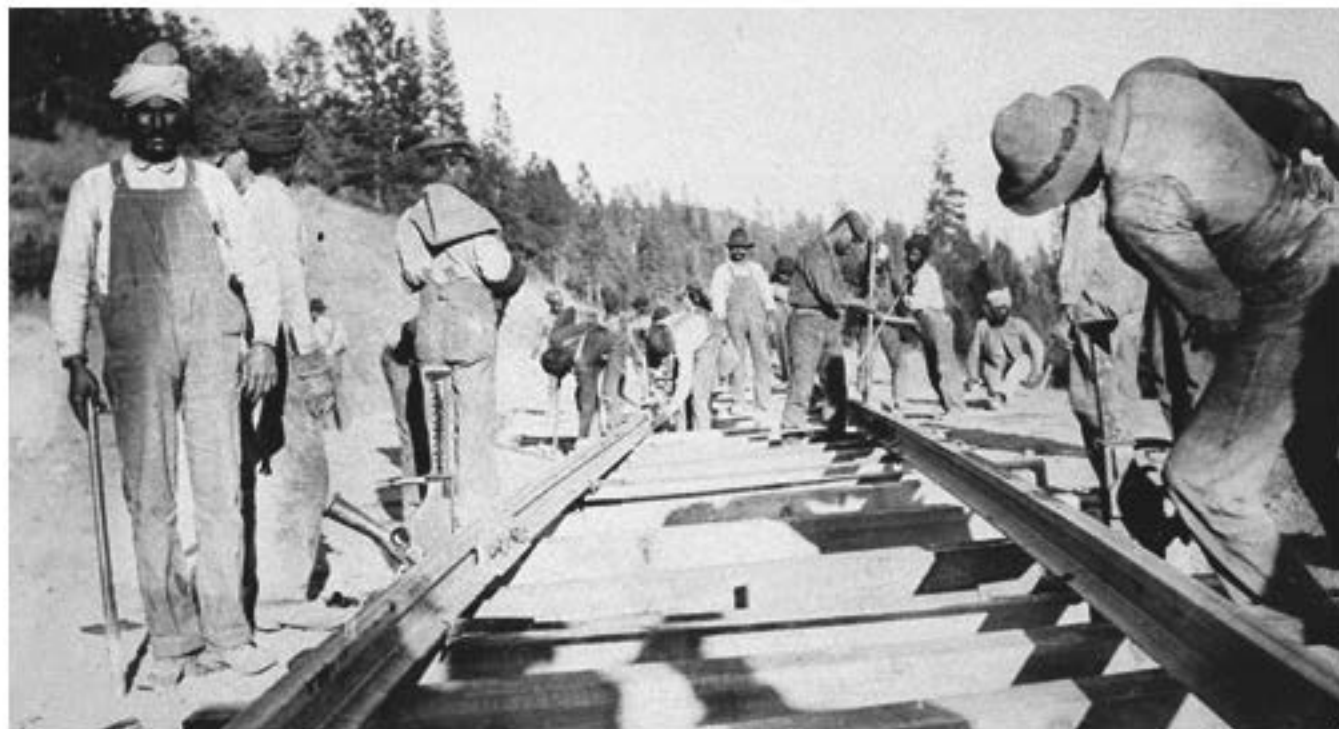
A crew laying track
