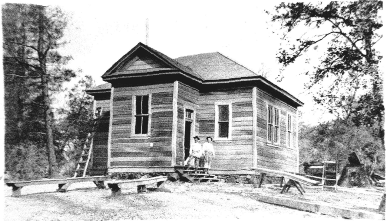
Brothers Oliver Lunt and Alfred Busch rebuilding the Concow school after the first school burned in 1907. Pictured is the backside of the new school. This second school burned in 1939
