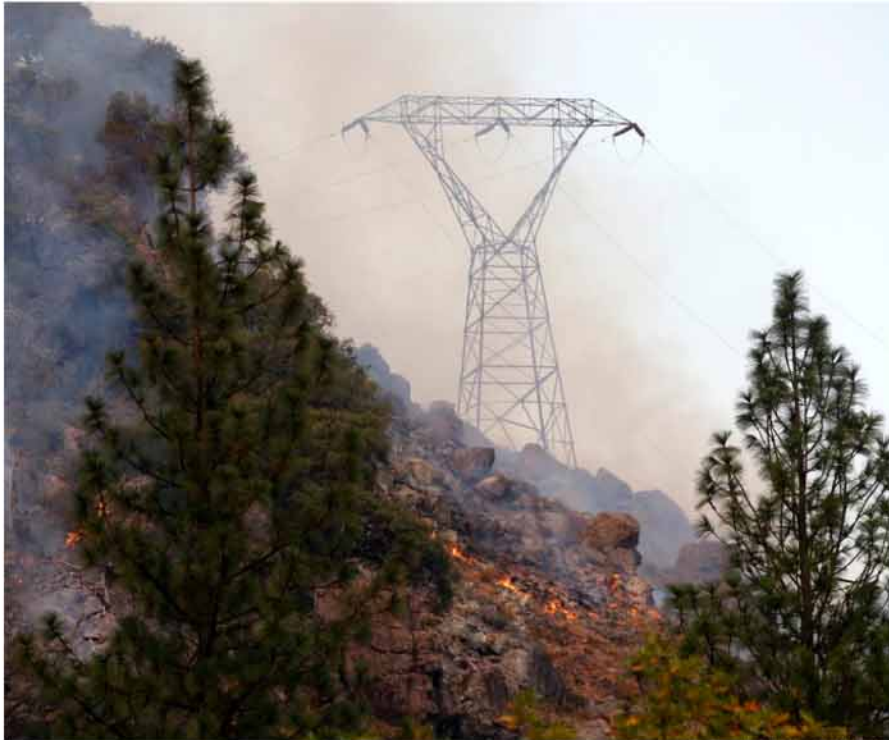
Fire smolders under high voltage towers in Pulga near the reported start of the Camp Fire blaze that destroyed the town of Paradise.
