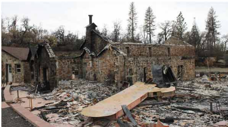
The historic Rock House located on Yankee Hill on Highway 70 was a familiar site to anyone traversing the Feather River Canyon. It was built in 1937 using horse and wagon to locally source the rock. The walls are 18 inches thick and are all that's left of the main structure. The owners lost not only the business, but also their home as the Camp Fire swept through the area the morning of Nov. 9, the day after the fire began. Photos by Victoria Metcalf
