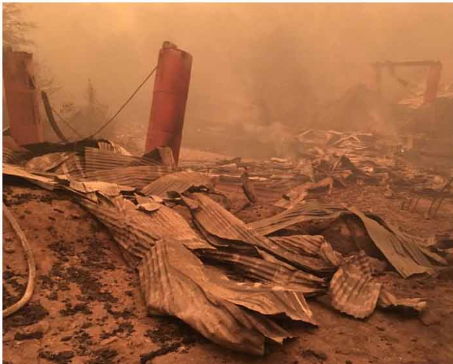
Nothing but supports remain from the historic wooden Honey Run Covered Bridge in Butte Creek Canyon on Friday after the Camp Fire roared through the canyon. The bridge, listed on the National Register of Historic Places, was built in the 1890s.
