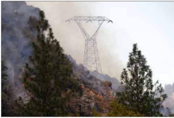
KARL MONDON — BAY AREA NEWS GROUP Fire smolders under high voltage towers in Pulga near the reported start of the Camp Fire.
