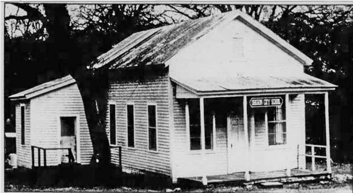
Everything from the front porch to the chimney of the Oregon City schoolhouse had to be fixed
