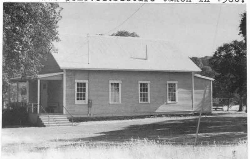
Cherokee school after top story was removed. Picture taken in 1960.
