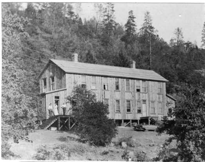
Hospital at Camp 6 along Highway 70
