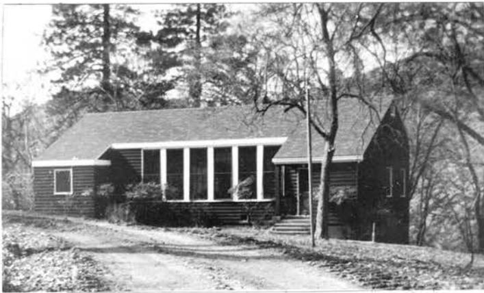
Las Plumas School. Feather River Canyon. Now covered by waters of Oroville Dam. Early bridge across West Branch at Nelson Bar.
