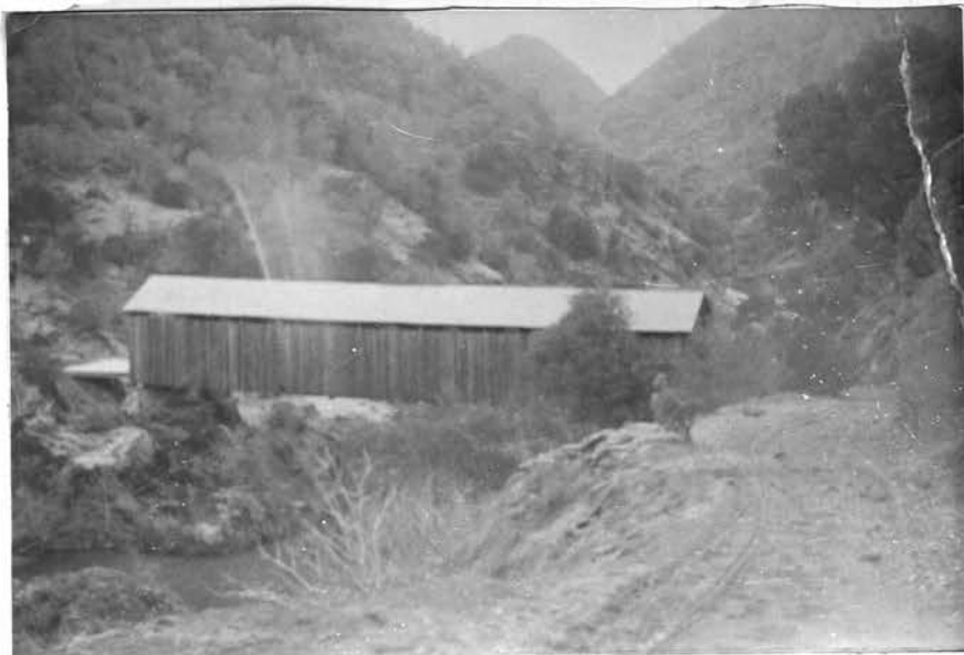
Nelson Bar bridge.
