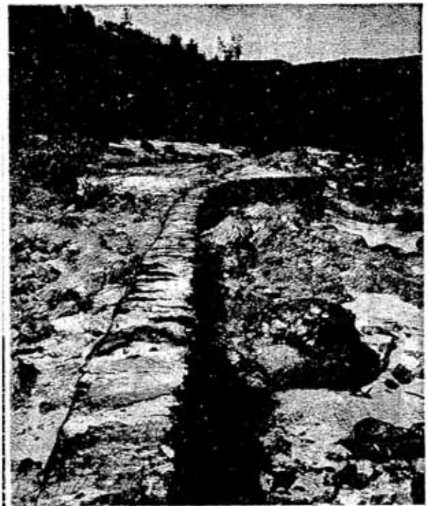
The wall is four feet wide at the top, 12 feet at the base. In some places it is 20 feet high.
