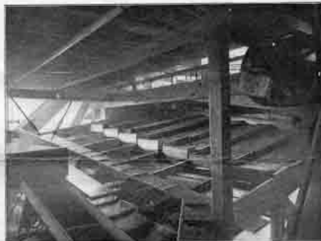
THE GOLD-SAVING TABLES OF A CALIFORNIA DREDGER.
