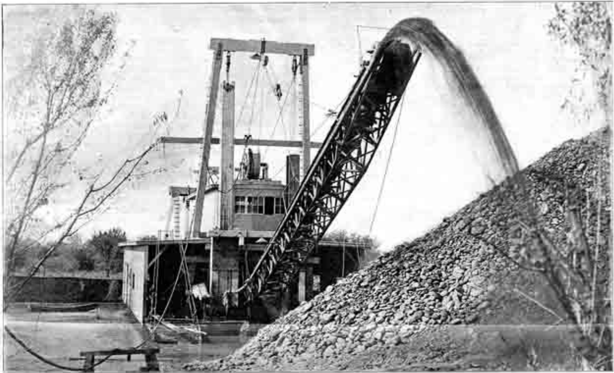
THE DREDGER "INDIANA" PROVIDED WITH A CONVEYOR AND AN AUXILIARY SAND PUMP.
