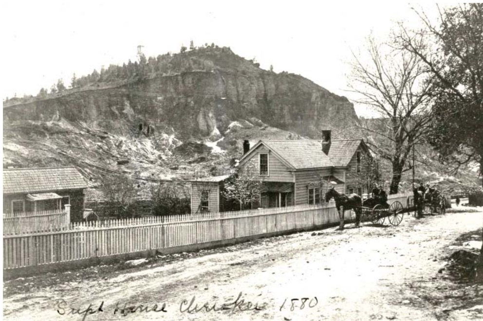
Cherokee Mine Superintendent's House
