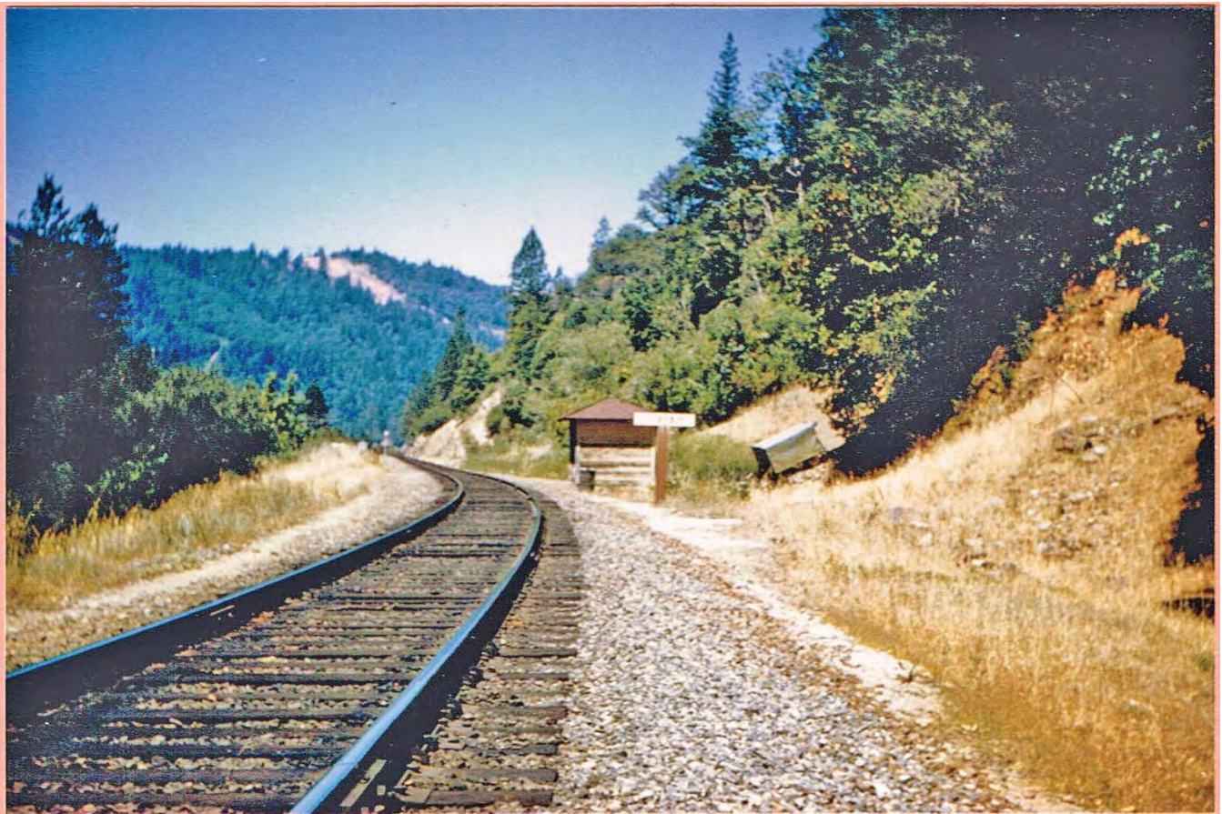
Isaiah Stop 1962, community was up the hill, see small tram car to transport goods to the community.
